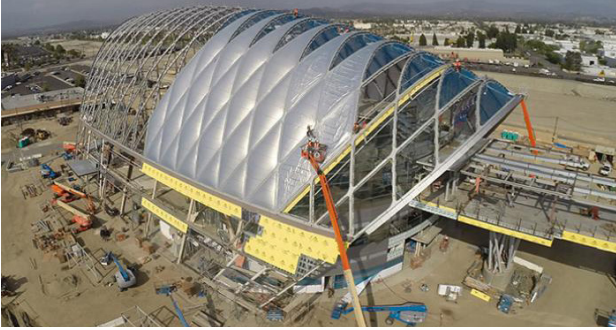
Figure 57: ARTIC Construction Photograph
