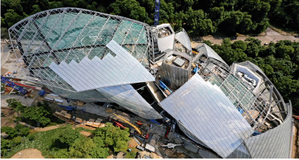
Figure 41: Fondation Louis Vuitton Glass Panel Installation
