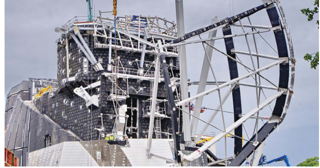
Figure 42: Fondation Louis Vuitton Glass Sail Frame Construction
