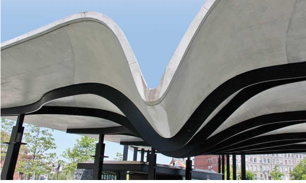
Figure 28: Boston Harbor Park Pavilion. Digitally Fabricated Formwork & Cast-In Place Concrete Construction
