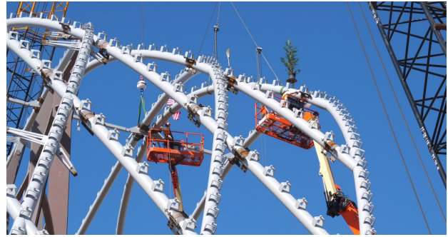
Figure 59: ARTIC Steel Erection Photograph
