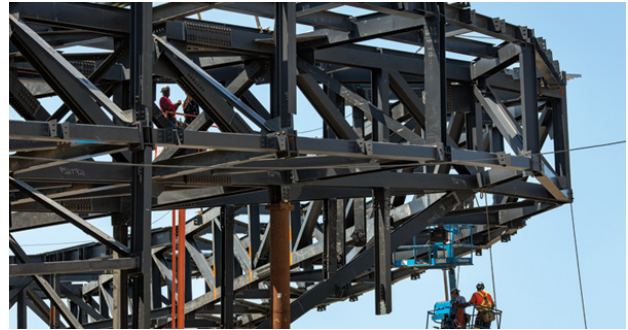
Figure 52: Barclays Center Canopy Structural Framing Photograph
