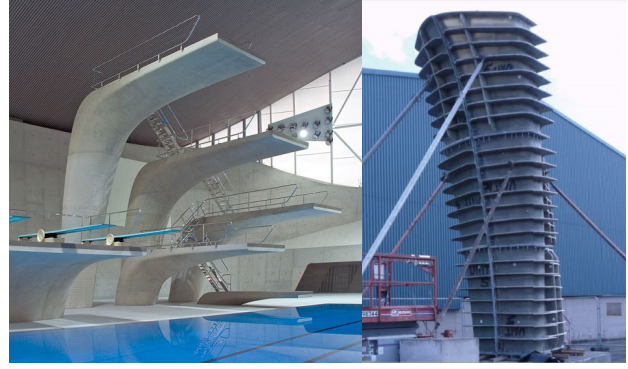
Figure 29 Olympic Diving Platforms, London 2012, Form created by 5-axis CNC and Glass-fiber Reinforced Polymer Formwork for Precast Concrete Construction
