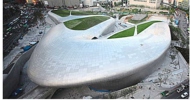
Figure 47: DDP Exterior Photograph
