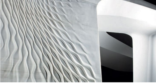
Figure 34: Waterjet CNC Fabricated Stone Wall Design by ZHA
