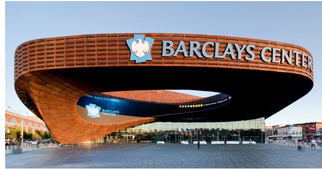
Figure 51: Barclays Center Exterior Photograph
