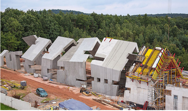
Figure 26: Mausoleum in Michniow, Injection Forming Concrete Construction
